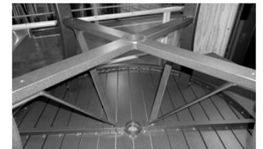
Install (2) Carriage Bolts with Flat Washer and Locking Nut through the top side of the Table Support Brace and into the Leg Support Brace (4) places.
